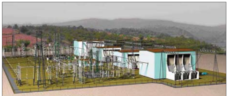
Fig. 5: A computer-generated illustration of an 800 kV converter station.
