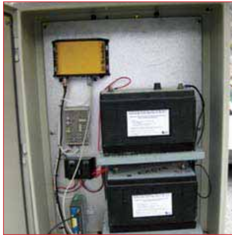
Figs. 7 and 8: The GPS receivers and wireless access points are powered by solar power.
