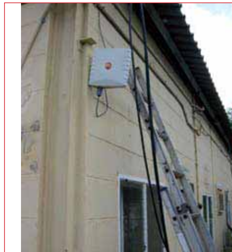
Fig. 5 and 6: Directional antenna at TIM installation 2,4 GHz, 15 DBi gain antenna 30° x 30° beamwidth.
