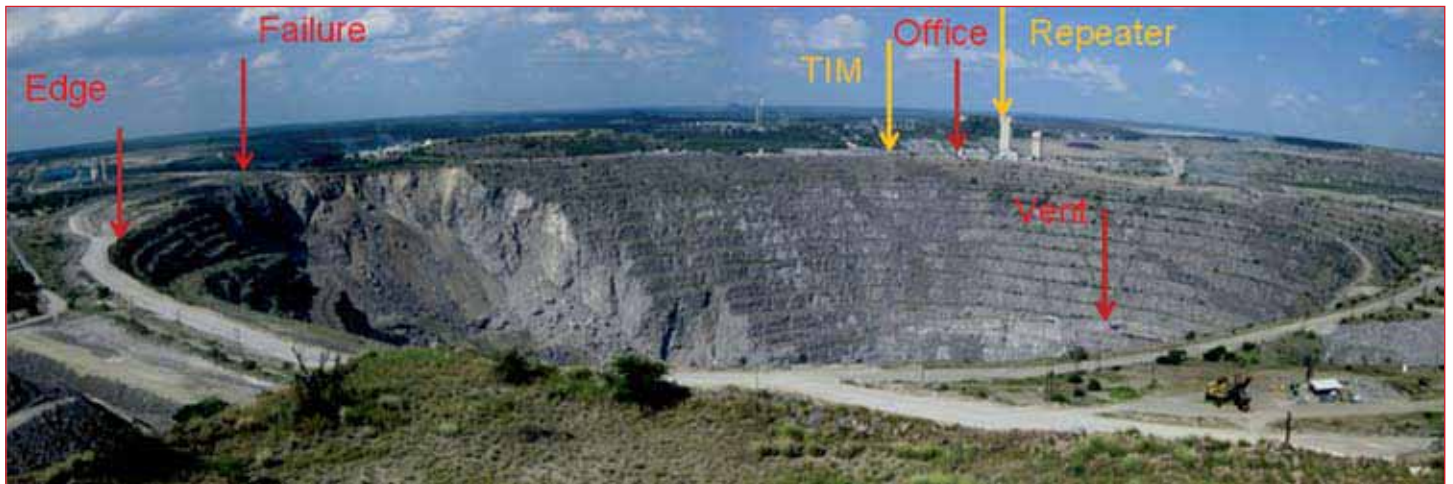
Fig. 3: The four stations transmit the GPS data to a repeater station on the headgear of the mine.
