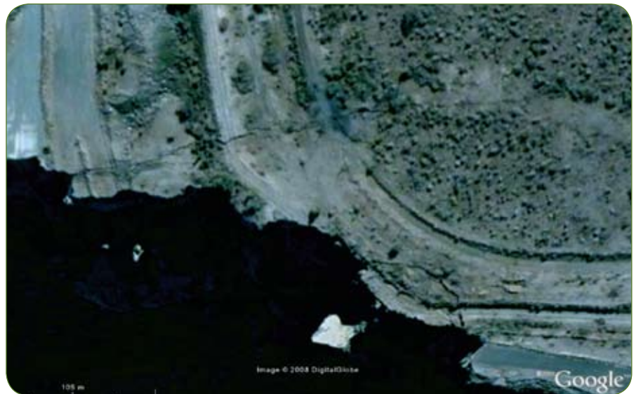
Fig. 2: Google Earth images close to the failure indicate that there is still ground motion.
