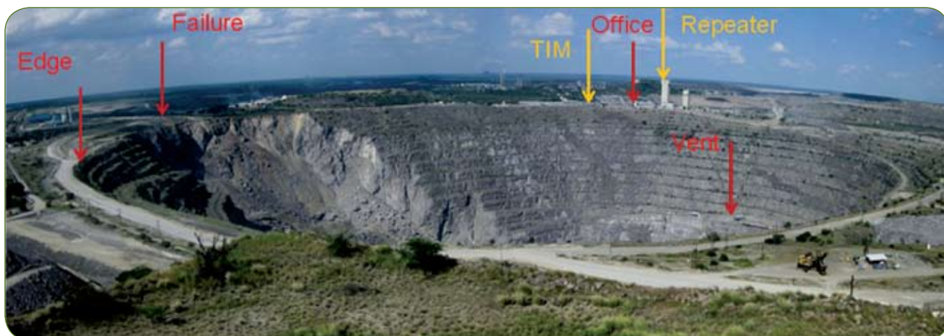
Fig. 3: The four stations transmit the GPS data to a repeater station on the headgear of the mine.
