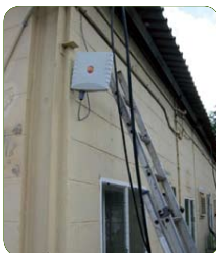
Fig. 5 and 6: Directional antenna at TIM installation 2,4 GHz, 15 DBi gain antenna 30° x 30° beamwidth.
